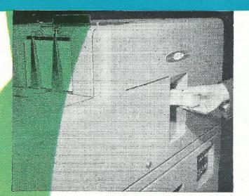
The card punch—at a speed of 100 cards per minute-will punch 64 decimal digits from the computer in any columns of the card, together with characters from the alpha/ numeric storage unit.
